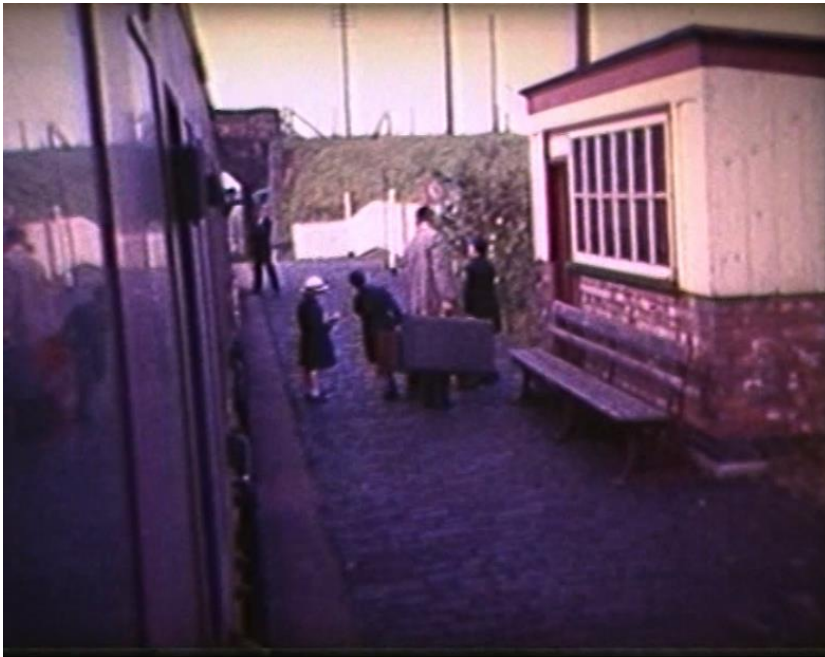
Hodnet's Southbound Platform. Station Road Bridge in Background
