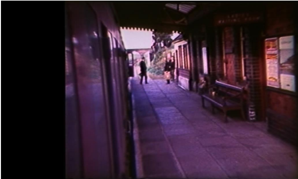
Tern Hill – Southbound Platform. The Station Masters House, not seen, survives - off to the right.
