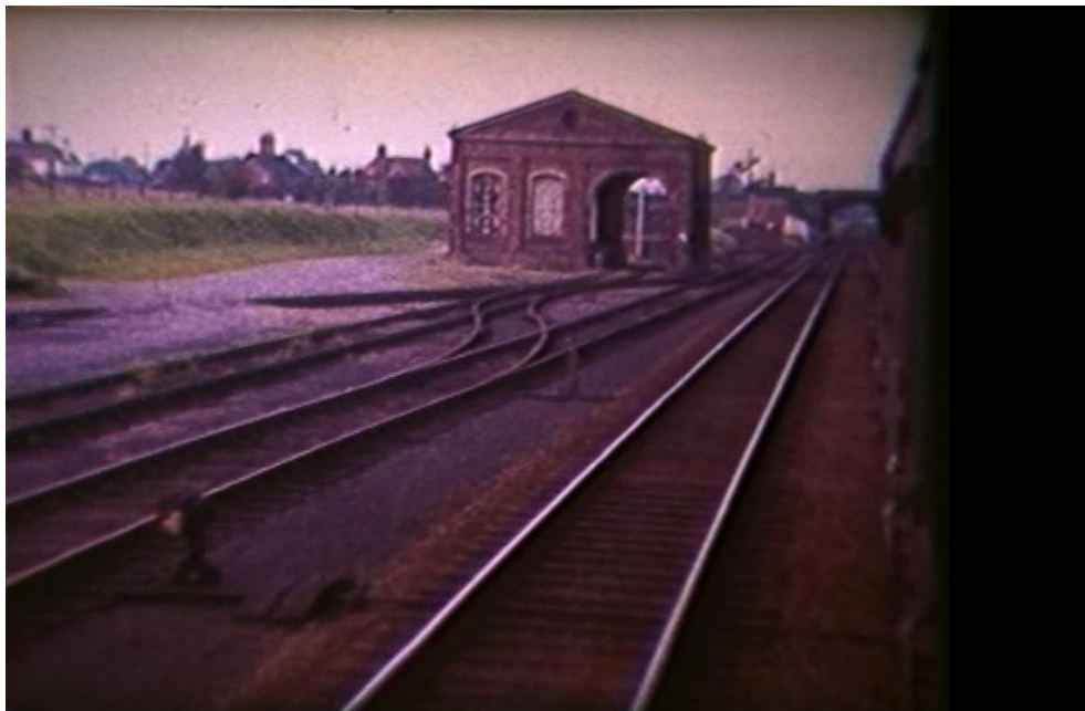
Hodnet's Goods Shed – Still Standing - Now Houses Supply Pumps for Shropshire Groundwater Scheme.
